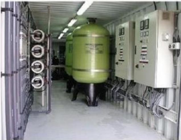
Containerized Seawater Desalination plant
