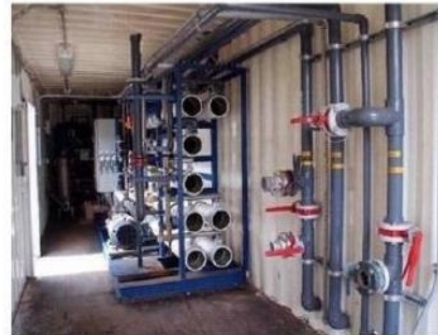
Containerized Seawater Desalination plant
